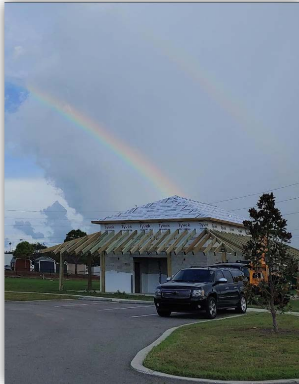
Restroom facility at Waterfront Park under construction in FY20.
